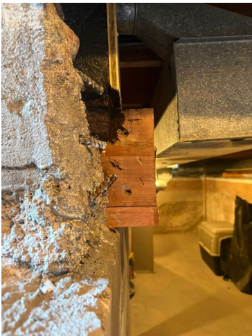
DURING - shoring and new ledger
