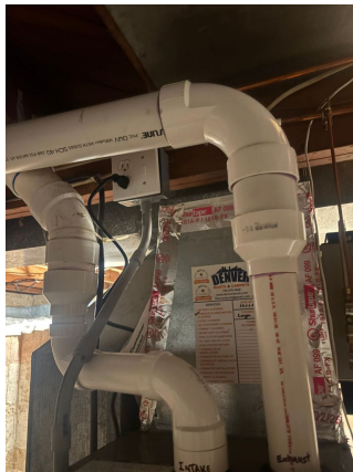
AFTER - new PVC intake and exhaust
