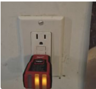
AFTER - GFCI tested
