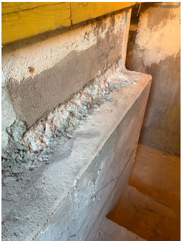
AFTER - rebuilt concrete at pocket
