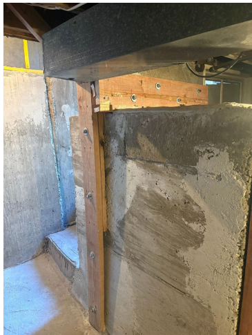
AFTER - rebuilt pocket and ledger
