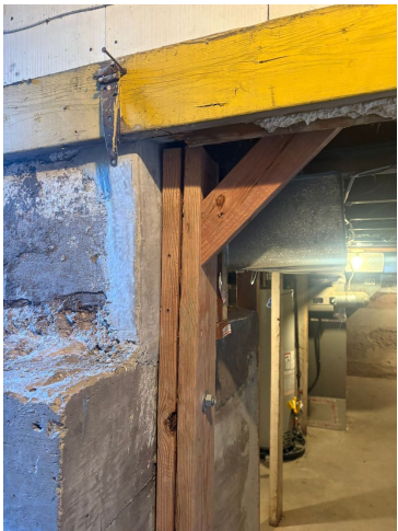
AFTER - completed repair, wall view
