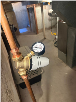
AFTER - new pressure reducing valve
