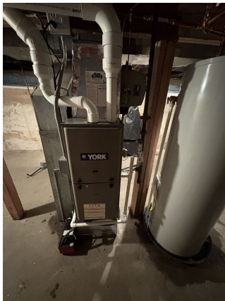
AFTER - new furnace and venting
